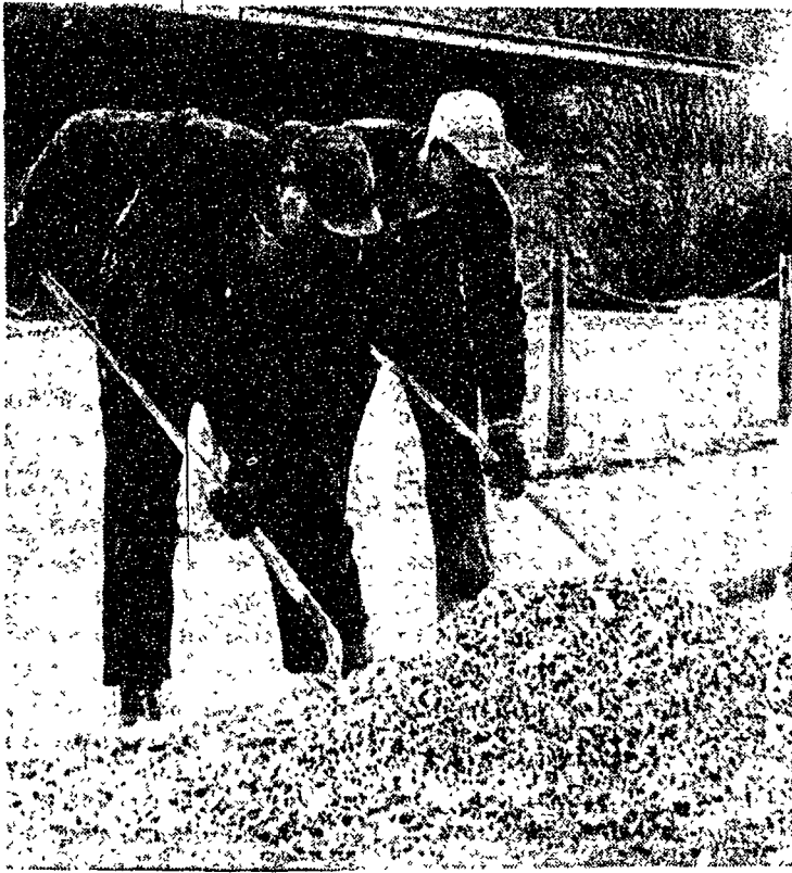
—Collegian Photo by Marty Scherr ASPHALT JUNGLE will expand when the workmen get through laying the foundation of gravel. The grass in front of Boucke and the HUB is now being removed to make way for asphalt walks.
