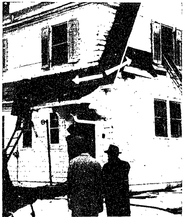
—Collegian Photo by Bob Thompson ALPHA FIREMEN douse stubborn flames that heavily damaged parts of home of H. Eugene Goodwin, director of the School of Journalism. The fire, believed to be started by faulty wiring, burned out two rooms and broke through three parts of the roof (arrows).
