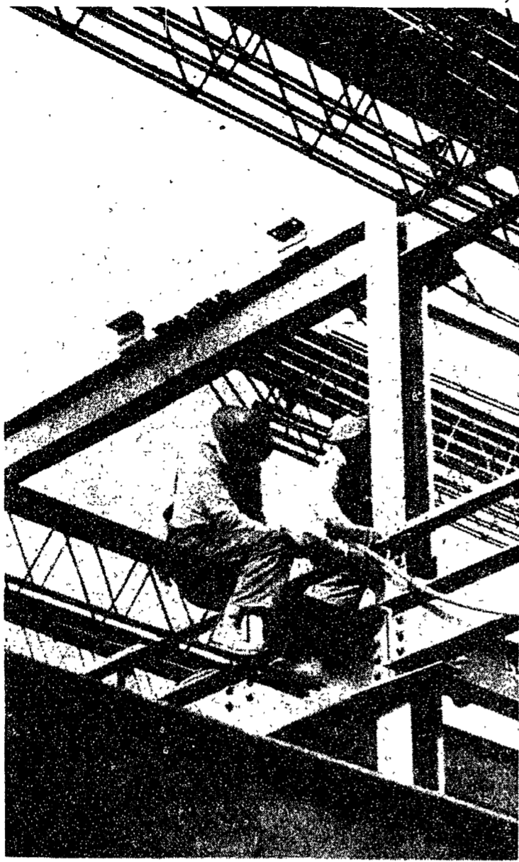
—Collegian photo by Bob Thompson SYMBOL OF THE FUTURE is the construction worker riveting the steel skeleton of one of the University's new buildings.
