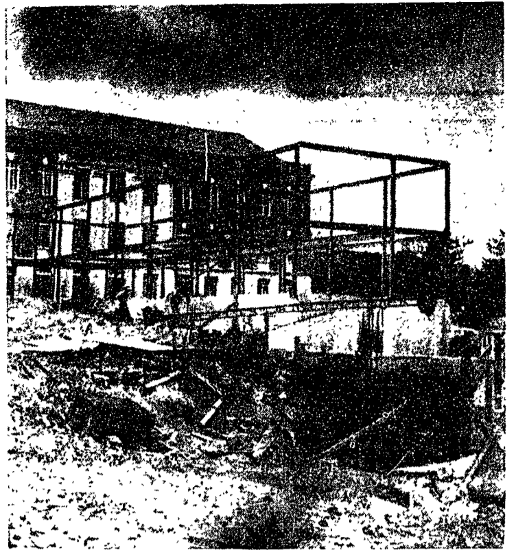
—Collegian photo by Marty Scherr TONS OF CONCRETE poured into these forms will form a base which will hoist the new home ec building onto its shoulders.
