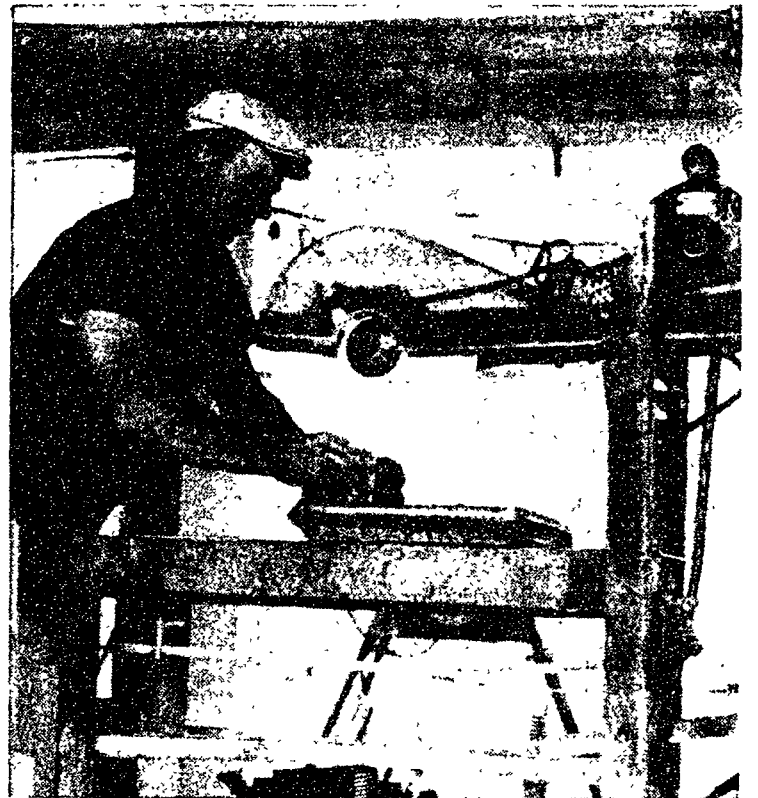
HOW MANY BRICKS could a brick cutter cut—if he had an electric saw with a diamond edged saw blade? That was the question asked by the photographer to the brickcutter (cutting bricks). But, the brickcutter (cutting bricks) couldn't hear him for the noise of the brickcutter (cutting bricks) was too loud.
