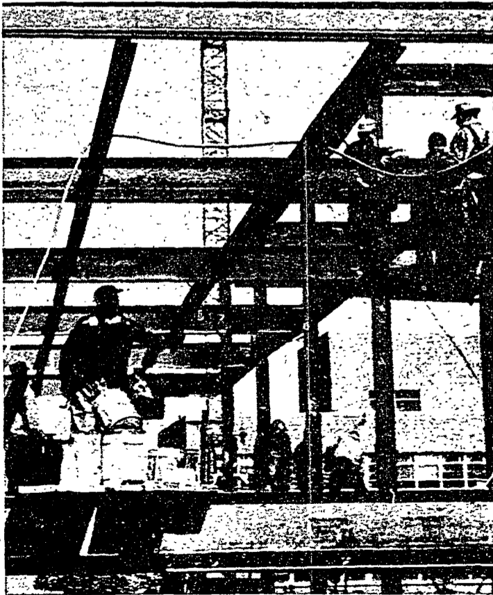
RAT-A-TAT-TAT—Riveters continue work on the first and second floors of the addition to the Foods Building on North Atherton Street.
