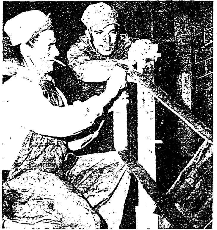
—Daily Collegian Photo by Marty Scherf TWO PHYSICAL PLANT WORKMEN, Oscar Lucas and Ed Siegfried, install a stairway railing in the Boucke Building, now receiving the finishing touches of construction.
