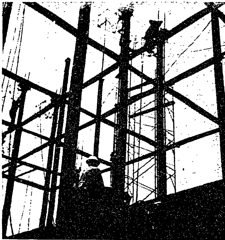
—Daily Collegian Photo by Marty Scherr WORKMEN use the new "lift-slab" construction method on the women's dormitories being built along E. College Ave. behind Simmons Hall.
