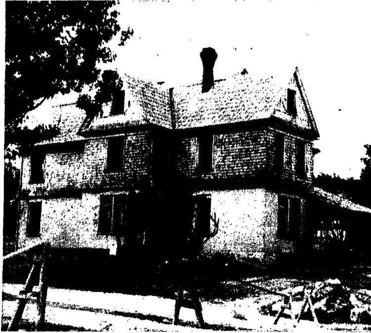
WORKMEN YESTERDAY started tearing down Maple Cottage in preparation for construction of the new classroom building. The new building will cost approximately $1 million 220 thousand and will house 63 classrooms and offices for over 110 faculty members. Of the 63 rooms, 22 will be furnished in the style of the nations of the western hemisphere.
