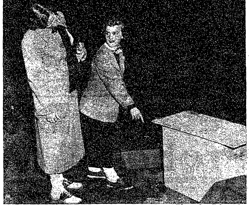
TWO UNIVERSITY COEDS Jean Geiger (left) and Carol Ann Huston examine the cornerstone meant for the Student Union building now under construction. Walter H. Wiegand, director of the physical plant, has said that no date has yet been set for the formal laying of the stone. The reason for the date being 1953 is that it marks the year when the building was begun.
