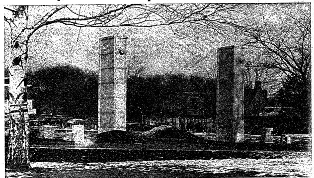
THE NEW CAMPUS GATEWAY, under construction at the intersection of Pollock road and U.S. Route 322, is nearing completion. The gateway consists of two 22-foot limestone pylons located to the north and south of the intersec-
