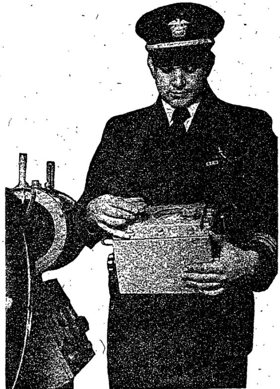
G-E engineers developed this portable steering unit which enables Navy ships to be steered from any of several widely separated strategic positions.
