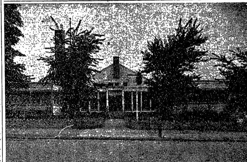
A POPULAR CENTER of student activities since its opening in the Fall of 1948, the Temporary Union building will again be open for the use of summer students. Formerly a USO center in Lebanon, the TUB was purchased by the College for use until a permanent Student Union building is erected.
