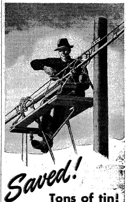
For years telephone cables have been spliced in a very satisfactory way. But the solder joint contained 40 per cent war-vital tin.
