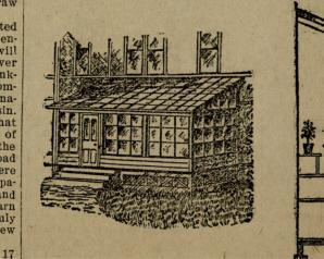
While most greenhouses are expensive to build and maintain, it is possible for an amateur to have one at small expense, as an addition to the dwelling. Hotbed sashes cost from \$3.25 to \$3.50 each, and measure 3x6 feet. If steam or hot water heating cannot be provided from the house, an oil stove will maintain a high enough temperature. temperature.
