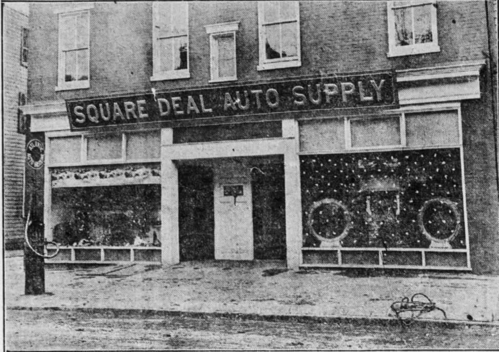
The above illustration shows the new quarters of the Square Deal Auto Supply Company at 1418 and 1420 North Third street. The entire first floor has been devoted to the display of accessories and motor equipment. This firm was formerly located at 1408 North Third street and few doors below the present location.
