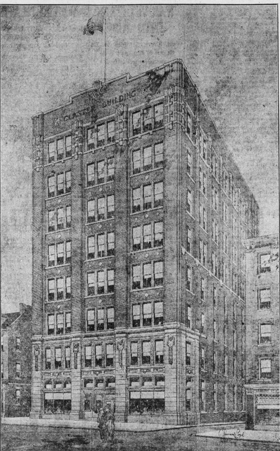
The work of remodeling the old Board of Trade Building, recently purchased by Henry C. Claster, is being rapidly pushed. This building, which will be eight stories in height, will be used by the State for office purposes. Howard Lloyd is the architect. The building will have a reinforced concrete frame. Gray tapestry bricks are being used on the exterior with Indiana limestone being used for trimming purposes. It will be equipped with the most modern devices throughout. There will be the latest in fire escapes, metal sashes and other safety devices. The building will be equipped with two passenger elevators and will have one large metal stairway.
