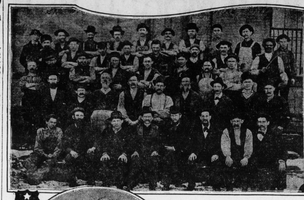
The upper photograph shows the company's employees in 1878. The lower shows W. O. Hickok, founder of the company.
