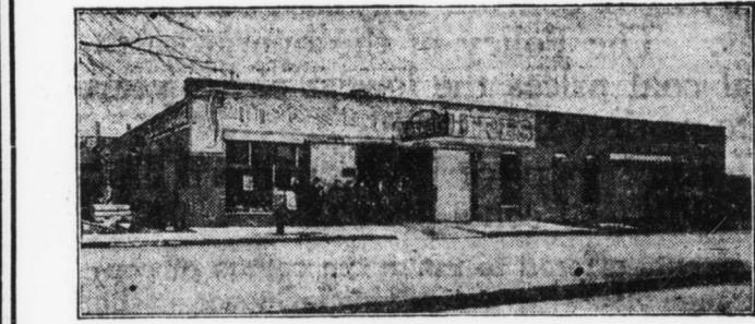
BLACK'S GARAGE Harrisburg, Pa., Feb. 26, 1919.
