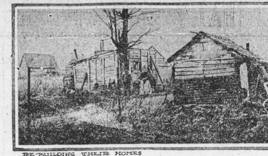
RE-BUILDING THEIR HOMES No more will the quaint built houses of French villages greet the eyes of the world tourists. The terrible destruction wrought by the Hun in northern France left the region desolate. With the withdrawal of the Hun army, French peasants immediately began the work of reconstruction. Due to the lack of material, everything possible was used in building shelters, with the result shown in the photograph. In the course of a year or two the villages will, no doubt, be rebuilt upon a modern lines, but the quaint architectural lines of centuries ago will be missing.
