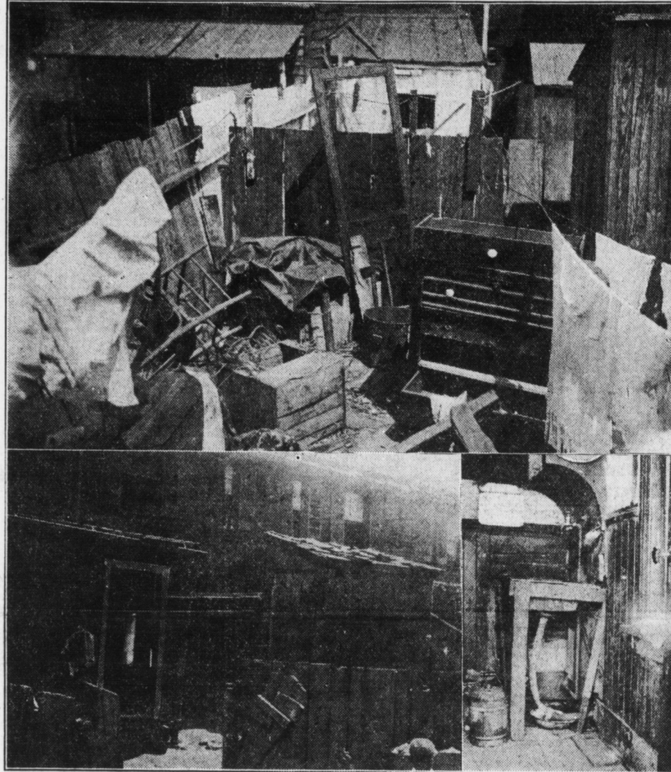
These photographs were made by a Telegraph staff photographer in the lower end of the city on Saturday. The sink in the picture has no trap; it leaks on the kitchen floor; the roof of this room hangs, the chimney is a firetrap and the outside toilet opens almost into the kitchen door; the plaster is falling off and the floor is rotting. The other etchings speak for themselves as to the need of improved housing conditions in the city.
