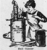
as illustration, will help you. It is made of 28 gauge galvanized steel, 21 inches high, 12 1-2 inches in diameter. Canning capacity, 12 one-quart fruit jars of any make or style.
