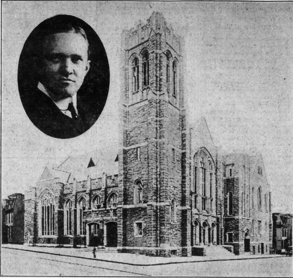
Messiah Lutheran Church, now one of the finest structures in the city, is to be formally turned over to the congregation to-morrow. The cut shows the Rev. H. W. A. Hanson, pastor, under whose direction the edifice was erected.
