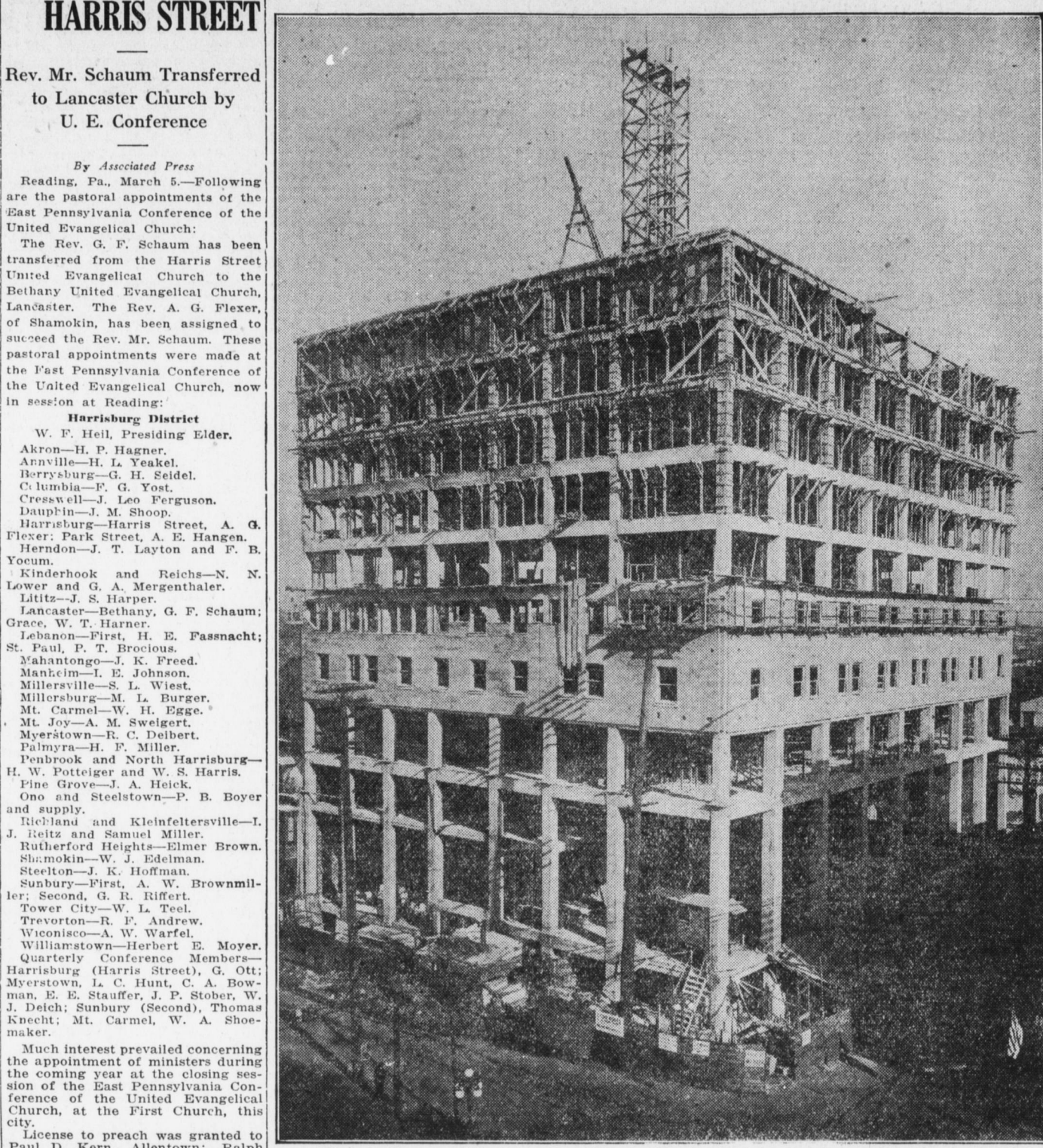
Work on the new million-dollar Penn-Harris Hotel is rapidly progressing, under the efficient direction of E. A. Johnston, construction superintendent, and R. B. Hawes, architectural superintendent. Concrete is now being laid on the tenth floor and forms for the roof are being constructed. The roof will be erected in a few weeks.
