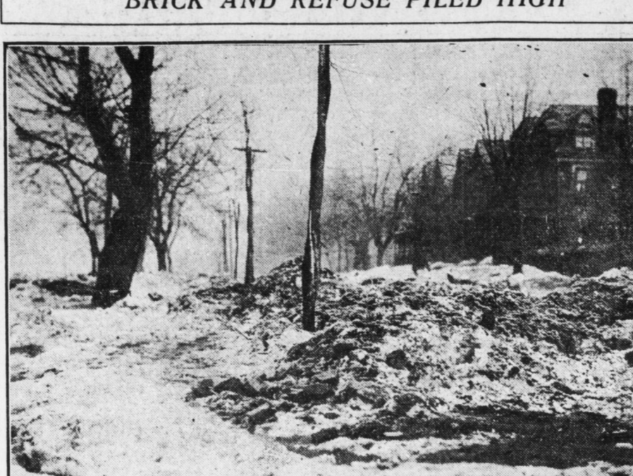
A pile of broken bricks and other refuse in River Front Park, just north of Calder street, dumped there in violation of park department rules, is shown above.
