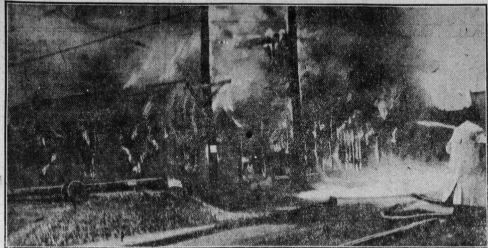
VIEW OF BUILDING JUST BEFORE IT COLLAPSED
