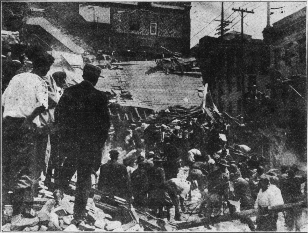
The photograph was snapped immediately after the collapse of the Underwood building which carried all in it into the excavation for the Penn-Harris hotel. A few minutes after the wreck hundreds were searching through the ruins for three girls reported to be underneath the tons of brick and mortar.
