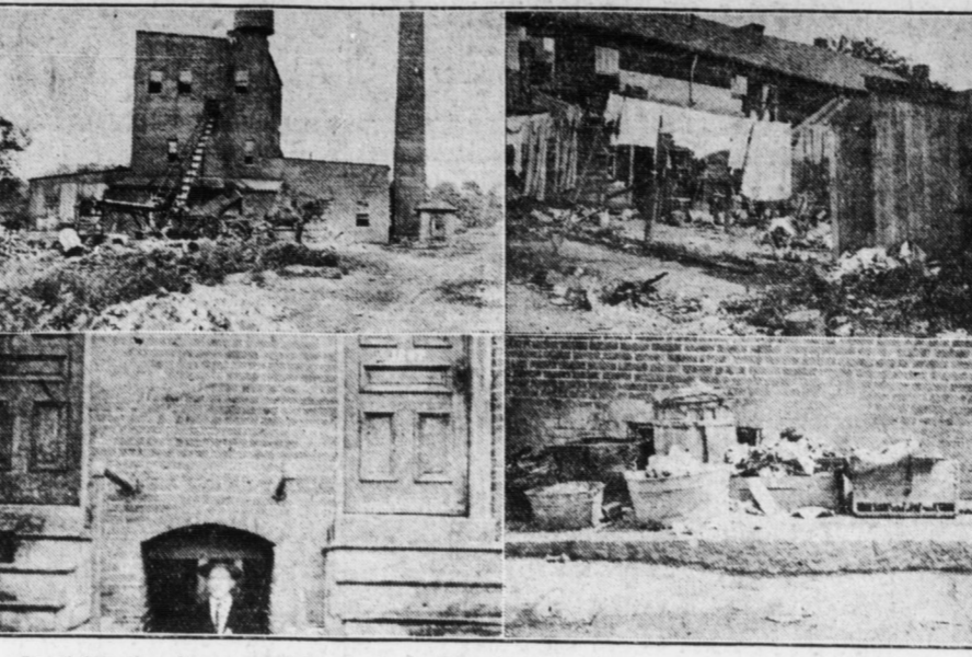
In giving the city a complete report on the ash and garbage survey, with recommendations for the establishment of a municipal ash bureau, Tribus and Massa, the engineers making the investigation, included a number of photographs showing conditions as they exist in Harrisburg. Some of these are reproduced above. On the left at the top is the present plant of the Pennsylvania Reduction Company, where all garbage is taken. To the right is a view of yards in the vicinity of Cameron and Cumberland streets. Below on the left is a "subway" near Seventh and Verbeke streets, less than three feet in height. Collectors are compelled to pass through it to gather ashes and refuse in yards in the rear, a condition which should not exist, the engineers say. To the right is an accumulation of ashes and rubbish in boxes piled in the street.
