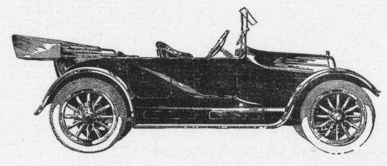
4 cylinder en bloc motor 3%" bore x 5" stroke 4-inch tires, non-skid rear Cantilever rear springs Streamline body
