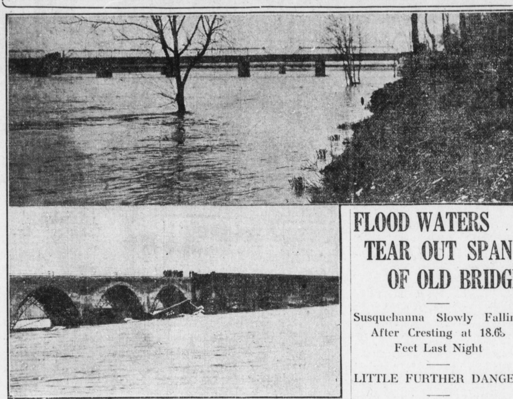
The upper picture shows how the flood waters of the Susquehanna have hid from view the city's Front Steps and River Wall and how near the stream came to overflowing its banks. The picture below shows where the rush of water washed away a section of the old Cumberland Valley railroad bridge, now being dismantled.
