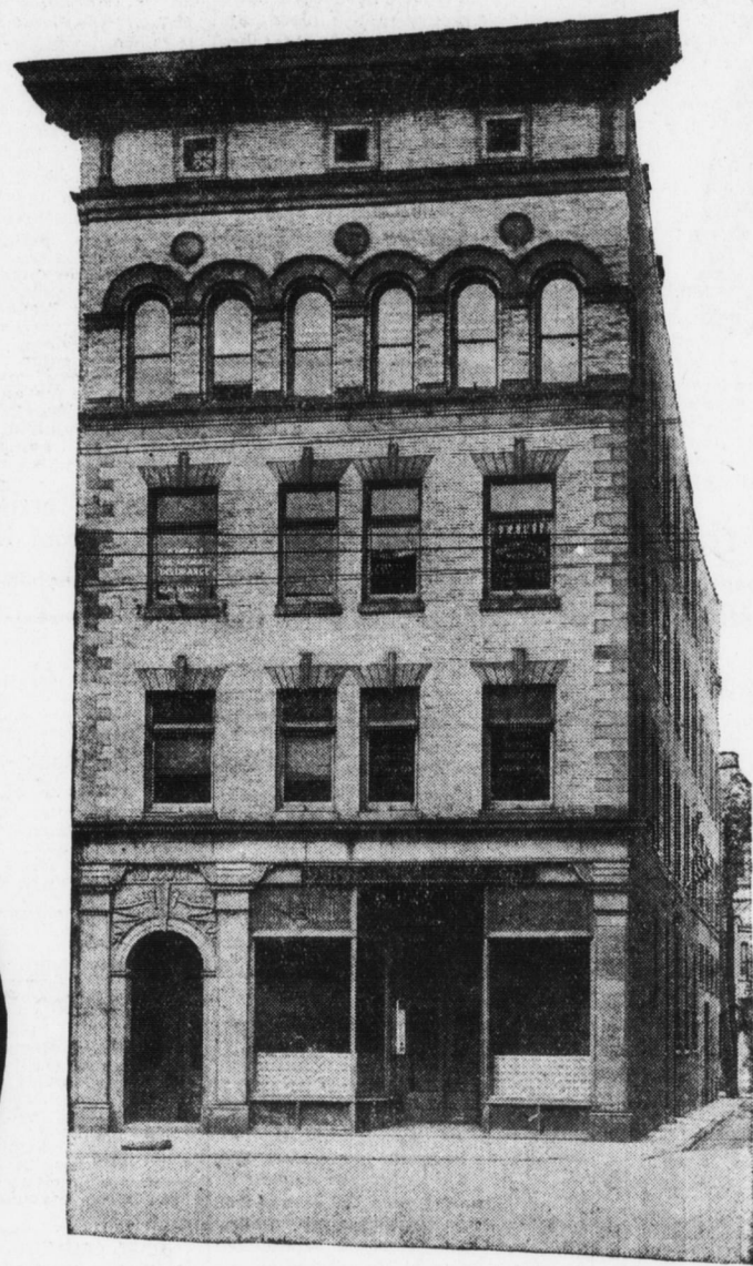
18 NORTH MARKET SQUARE Present Location of the Executive Offices.
