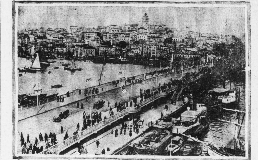
It is reported that a British submarine has blown up a portion of the famous Galata bridge, which spans the Golden Horn at its point of junction with the Bosphorus, and connects Stamboul and Galata, two of the most important sections of Constantinople.
