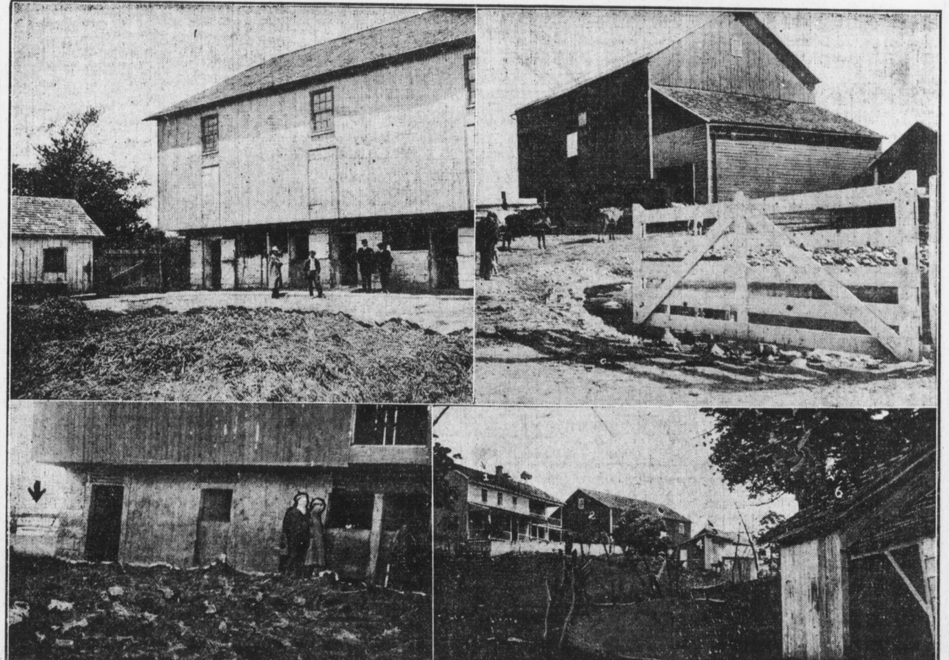
Lower left.—Barnyard on farm near Newville where manure covers the ground to a depth of more than two feet in some places. The arrow points to the trough where milk cans are washed, the water being drawn from a cistern which gathers rain water from the roof of the barn. One test made of the milk from this farm showed the presence of 30,000,000 bacteria to a cubic centimeter. Another test showed 60,000,000 in the same quantity. That milk is no longer coming to Harrisburg. Lower right is a scene on farm near Penbrook, where tenant at present is confined with typhoid fever. No. 1, shows the house; No. 2, the barn; No. 3, the pig pen; No. 4, the chicken coop; No. 5, the toilet; No. 6, the spring house where milk cans are washed and where the milk is cooled. All of the buildings, with the exception of the spring house are on the hill and drainage from these naturally finds its way to a little gully at the base. Much filth can be found in this gully which leads directly to the spring house. This producer, until he became ill, was one of the farmers who sold his milk to a big dealer in a nearby borough, who in turn supplies hundreds of Harrisburg families. Upper left.—Scene on a well kept farm near Shoop's Church. The manure is scraped away from in front of the barn. The interior of the structure where the milk is taken to be cooled and bottled. This farmer delivers his milk in the city himself. The little building to the left is the milk house. Upper right.—Farm near Newville. Only a few feet from the barn is a hole filled with water from numerous rains. The water is filthy and in this covey are permitted to wade before they are milked. The pond, which is a regulation malaria "park" has no outlet. Milk from this place is no longer being brought here.
