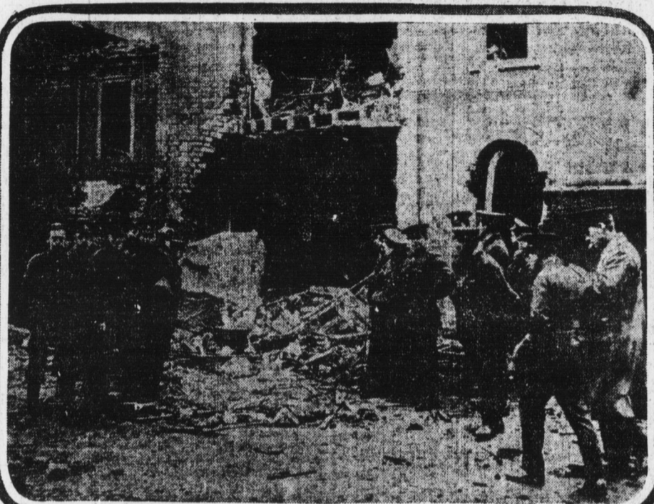
Damage done to buildings on St. Peter's Plain, Yarmouth, England, on the night of January 19, when a squadron of German Zeppelins dropped bombs on Yarmouth, King's Lynn, Sandringham and a number of other places in the vicinity.
