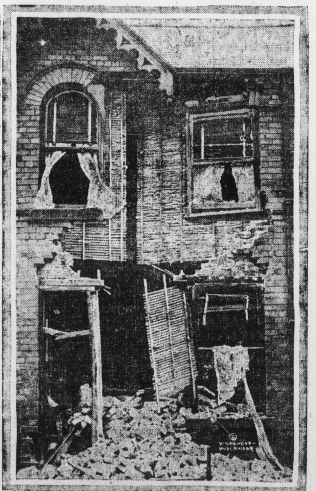
This building in Crescent, Scarborough, was torn open by the shells from the German warships which raided the east coast of England, December 15. One went through the roof, which was occupied at the time. So far as the information about it shows no one was killed, though several persons were injured. Many houses in Scarborough which were in line with the German shells show as much damage.
