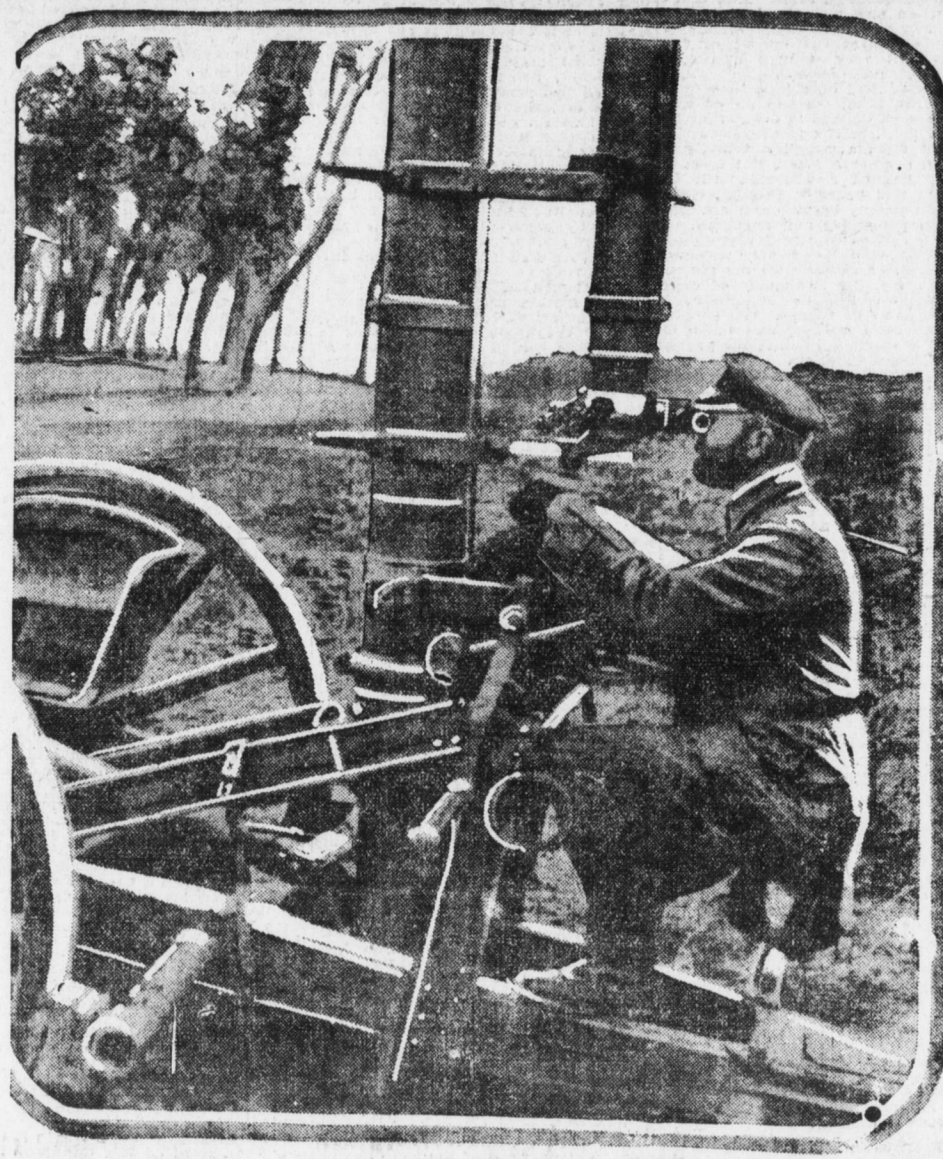
This German artilleryman is shown finding the range of the enemy's position by means of a newly invented telescope, similar in many respects to the periscope of the submarine.
