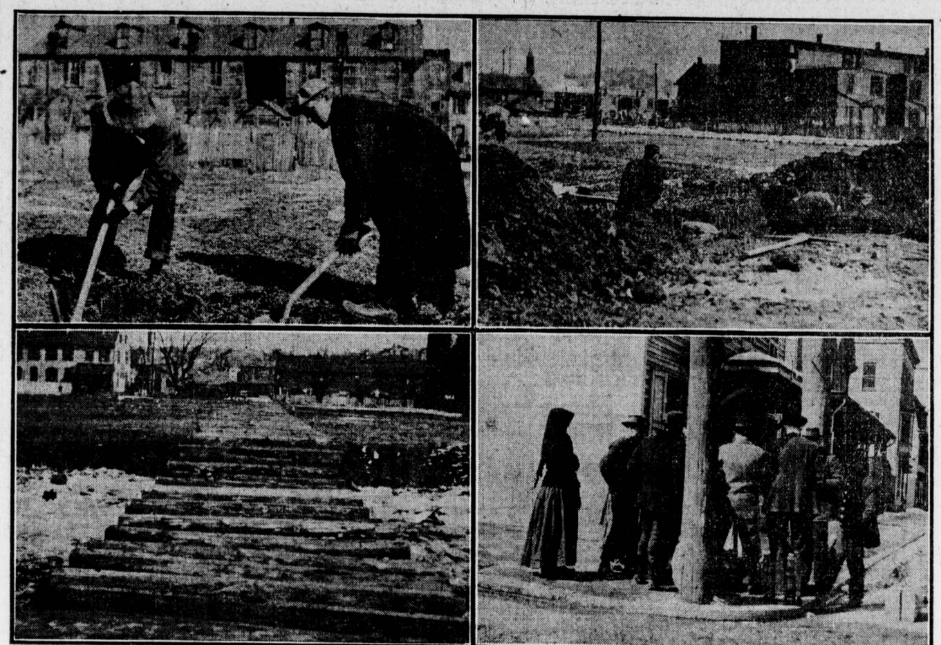
The Pennsylvania Steel Company yesterday broke ground for the mill extension work in the lower west side of Steelton which will wipe out at least fifty dwelling homes.
