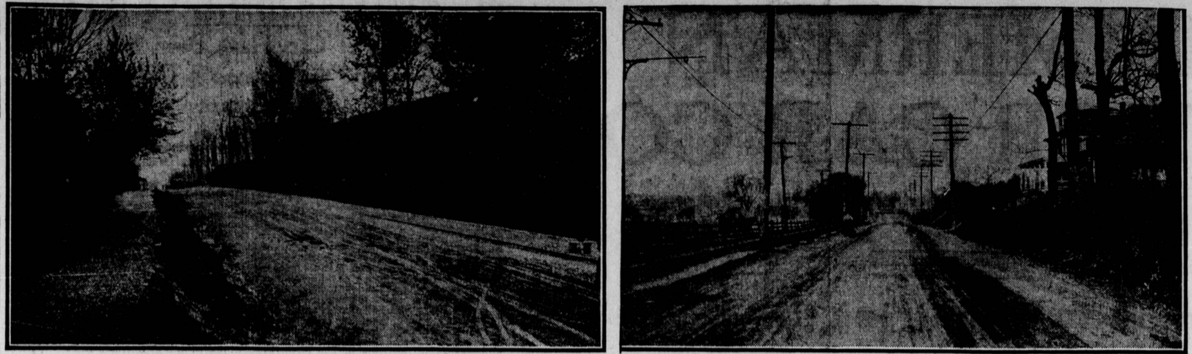
RESULTS OF PENNSYLVANIA STATE HIGHWAY DEPARTMENT IMPROVEMENT WORK IN THE VICINITY OF THE CITY OF HARRISBURG
