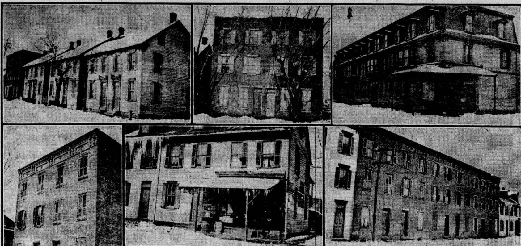
Photographs taken by a Telegraph photographer show various sections of the lower "West Side" of Steelton that will be razed by the Pennsylvania Steel Company to make way for extensive improvements at the plant in the near future. Fifty-one properties below Trewick street will be torn down, the residents of the properties having been given notice to vacate the premises within thirty days.
