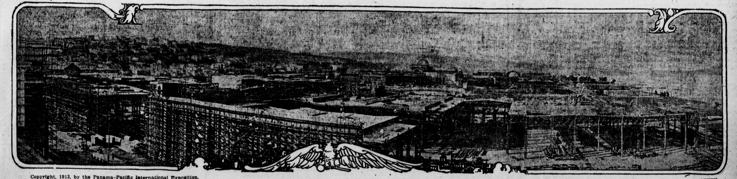
This photograph, taken from the roof of the huge Palace of Machinery, shows a part of the main exhibit section of the Panama-Pacific International Exposition after three months of actual construction upon the buildings here shown. Before the buildings could be erected an immense amount of preliminary work was accomplished. Great lagoons were filled in by suction dredges and more than eighteen months were spent in leveling and laying out the grounds and in preparing for the record-breaking work now under way.
