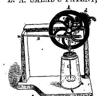
For Converting Rotary into Reciprocating Motion, and Vice Versa.
