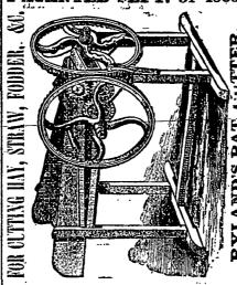
The merits of this machine consists in part, in the attachment of curved knives to the arms of the cutting-wheel, the shearto the arms of the cutting-wheel, the shearing cut across the mouth-piece, the great
