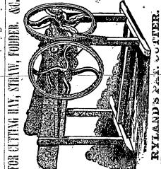
The merits of this machine consists in part, in the attachment of curved knives to the arms of the cutting-wheel, the shear ing cut across the mouth-piece, the great power and directness of the blow, by which reble the volume of material is cut, with less power than is required by any other machine; those combined with its durability and simplicity of construction, command public attention. Nothing liable to get out of order, but what a boy could remedy with pocket wrench.
