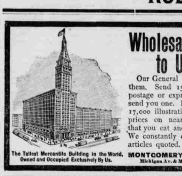
The Tallest Mercantile Building in the World. Owned and Occupied Exclusively By Us. MONTGOMERY WARD & CO., Michigan Av. & Madison St., Chicago
