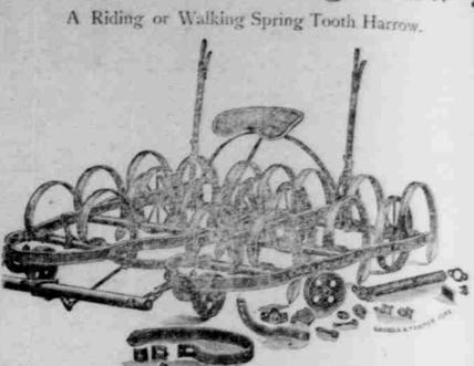
No dragging of frame on the ground. The lightest shaft. Willi clean itself of trash as easily as a hay rake. Runs as light with a man on as others do without a load.
