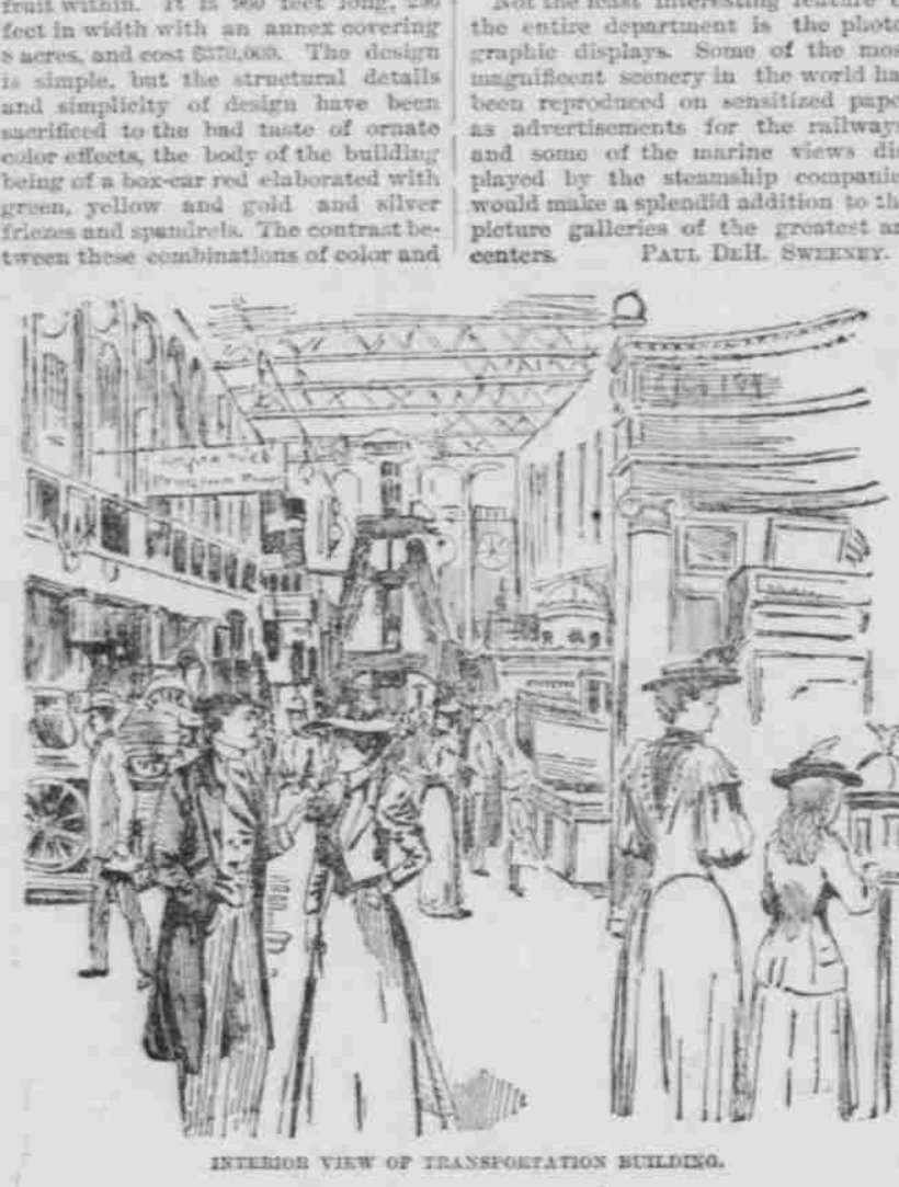
INTERIOR VIEW OF TRANSPORTATION BUILDING.
