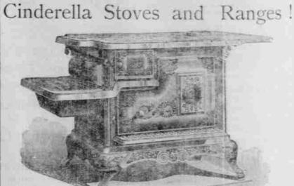
CINDERELLA-A. The best constructed Gooking Stove upon the marker, and GUARANTEED to give the satisfaction. The top is made in four pieces, so that it cannot crock. The long cost piece is cut in two and supported by a post, which prevents it from warping. It has an extra deep ash pit with balled ash part, and is we constructed that the ashes cannot accumulate under the grate, which is the chief cause of so many grates burning out.
