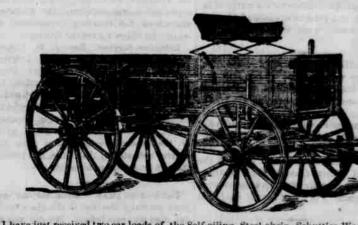
I have just received two car loads of the Self-oiling Steel-skein Schuttler Wagons, the most complete Western Wagon in the market for Road or Farm Purposes. On the latter there is a Rear Brake, to be used when hauling hay or grain, a something that farmers know the necessity of when hauling on hilly farms. Every part of the Wood-work of this wagon has laid in Stock three years before being worked up, insuring the work to be thoroughly seasoned before being ironed. Being the patentees of the
