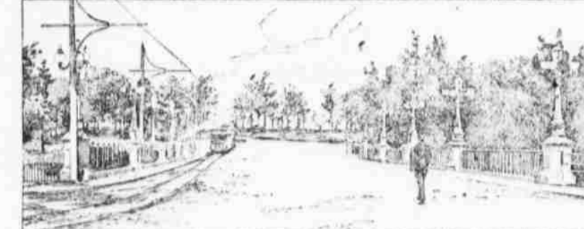
ELMWOOD AVENUE BRIDGE (Looking North).
