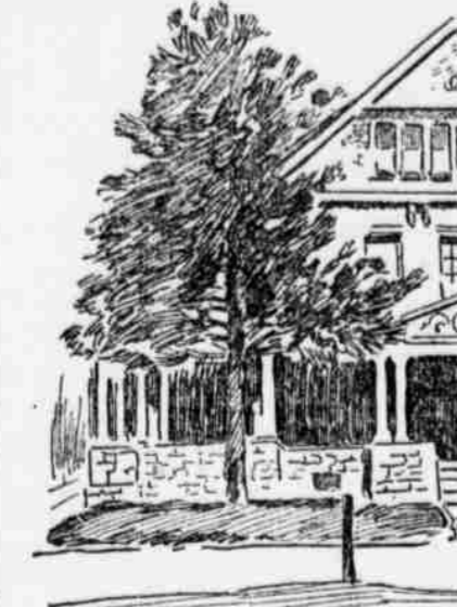
THE HOME OF L. E. WALLER. The Building That Was Wrecked by Dynamite on September 10, 1895.
